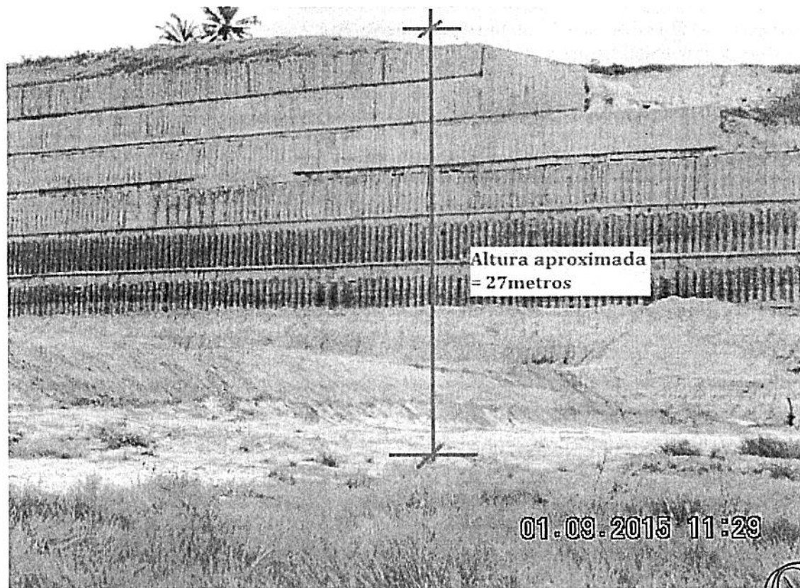
Foto 15: Execução da contenção de encosta no Terreno 4 Handwritten signatures and marks are present at the bottom of the page, including a large 'M' on the left, a signature in the center, and a signature with a circled 'A' on the right.
